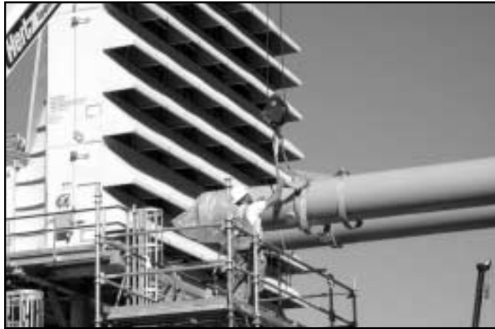
Ernest Stancil at work on the Pastoria project.
